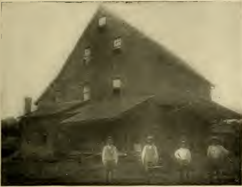
OLD VANDALIA FLOURING MILL.
